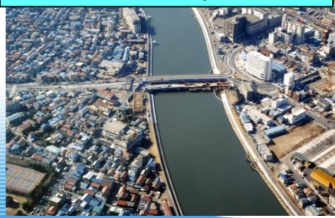
River channel improvement
